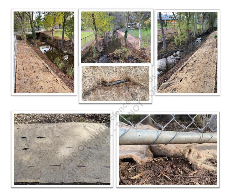
*Observation notes:* One bank of the creek with the jute weed matting . The groundsmen placed the mat into the ground using metal pegs.
